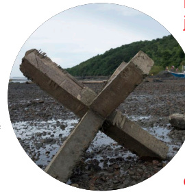
A concrete jackstone, part of an artificial reef.
